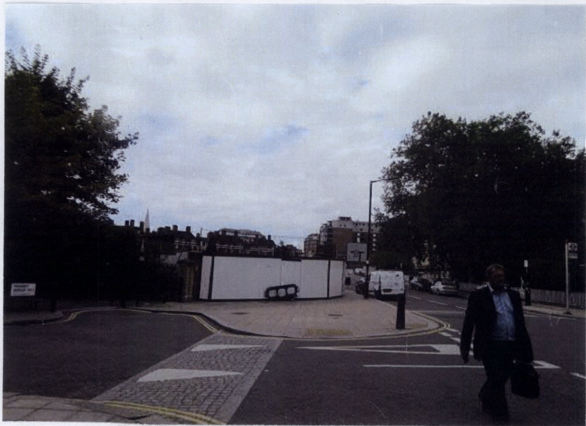
EBURY BRIDGE CENTRE, SUTHERLAND STREET, SW1
